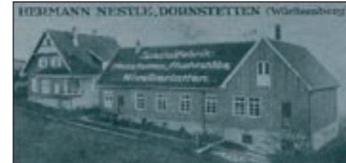
Company building in Riedsteige 1913
