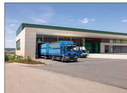
Nedo logistics center
