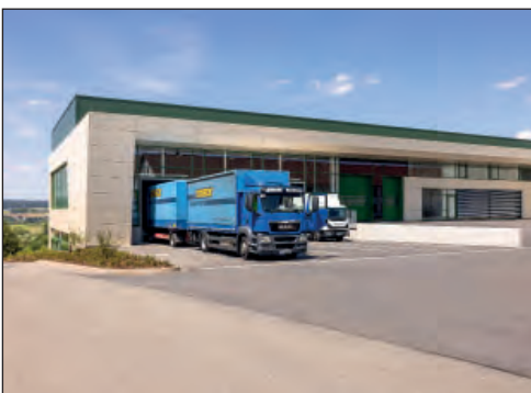
Nedo logistics center
