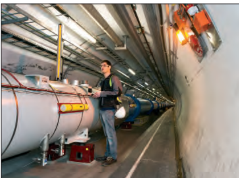
Nedo products in use at CERN
