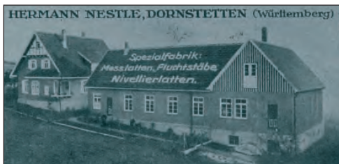
Company building in Riedsteige 1913
